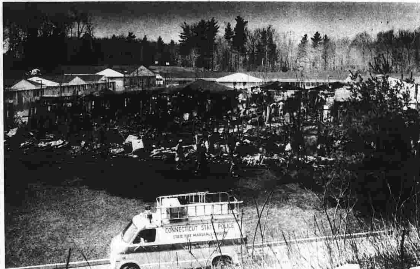
This is what was left Saturday afternoon of the Student Center building at Manchester Community College. The center, which also housed offices, the book store, and facilities for the food management program, was destroyed by an early morning fire. (Herald photo by Strempler)
