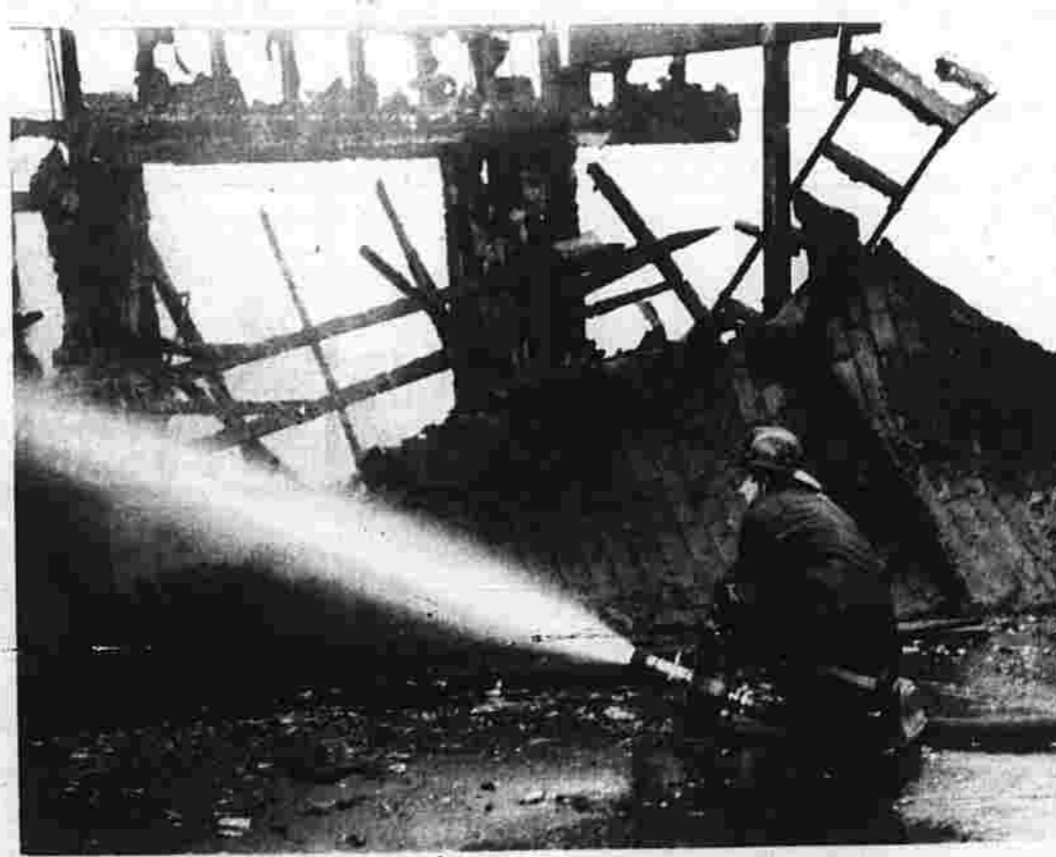
A wind-blown fire had gained a lot of headway by the time firefighters arrived at Manchester Community College Saturday morning. Fortunately the wind was blowing away from the mass of temporary buildings that make up the campus, and all were saved except the Student Center, which was destroyed. (Herald photo by Burbank)
